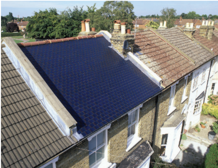
◀ FIGURE 9.17 Solar shingles look like traditional asphalt shingles but they are hooked into a home's electrical system.
