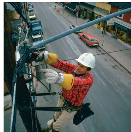
▲ People who work with electricity must be careful to use gloves made of nonconducting materials. Rubber, an excellent insulator, is often used for this purpose.
